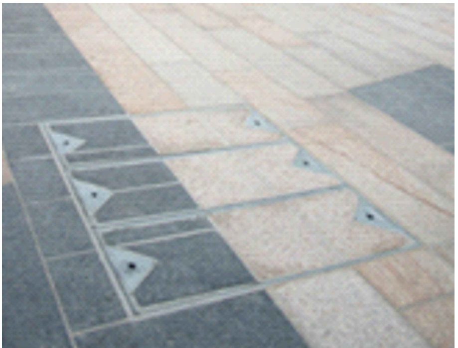
DETAIL B REPLACE ALL SINGLE LEAF RECESSED COVER AND FRAME WITH B125 FOR 75MM DEEP SLAB CPS2 TWIN LEAF FOR 600X600 AND CPS3 TRIPLE LEAF FOR 900X600 COVERS. TELEBLOC BY JONES OF OWESTRY.
