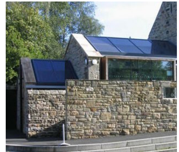
Above: PV installation integral to building design
