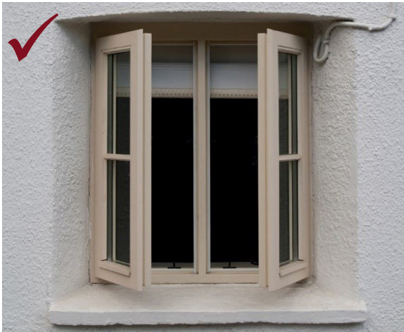
Above: timber opening casement painted window
