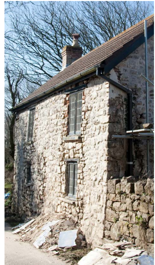
Above: Restoration works in progress, Middleton
