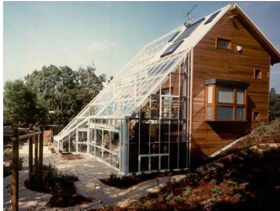
Above: BRE Integer House, Garston, Watford
