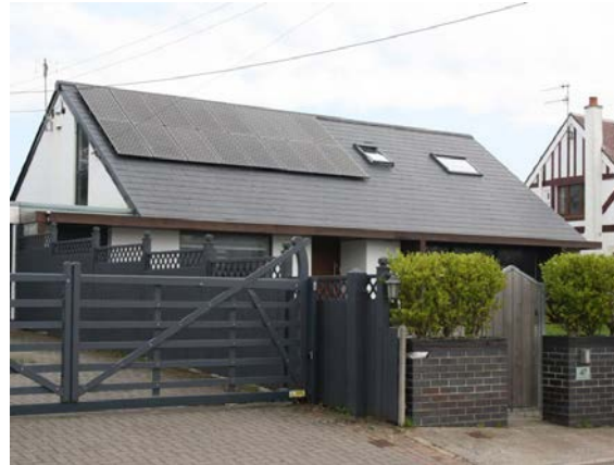
Above: Photovoltaics to roof, Southgate
