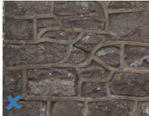
Inappropriate pointing to stone wall
