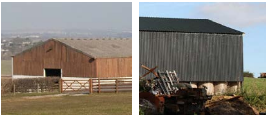
Above: illustration showing that using a double pitch reduces the overall building height
