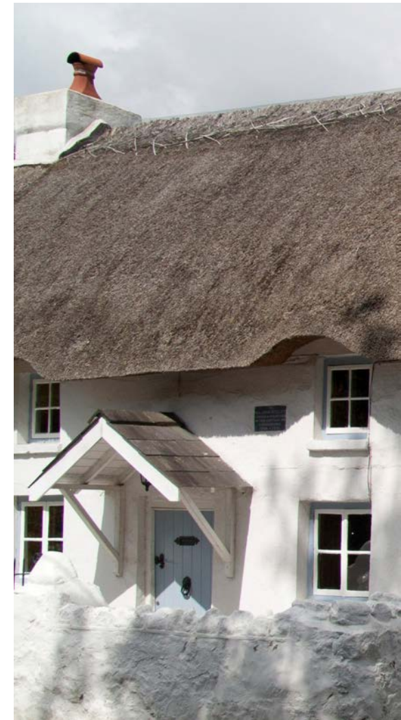
Above: The Nook, Oxwich: Grade II
