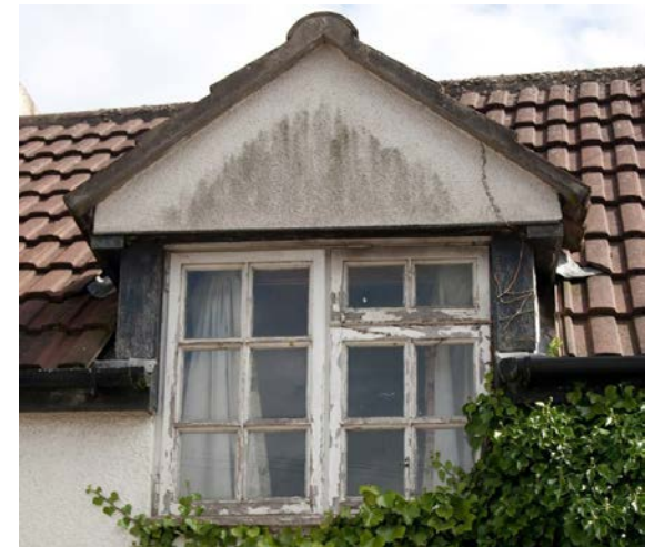
Below: poorly maintained windows can detract from the overall appearance of a building as well as allowing water to penetrate the structure.
