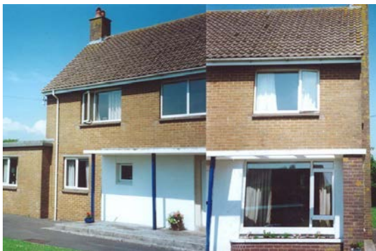
Above: before renovation
