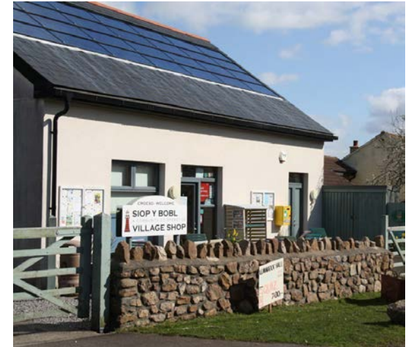
Above: PV installation Llanmadoc
