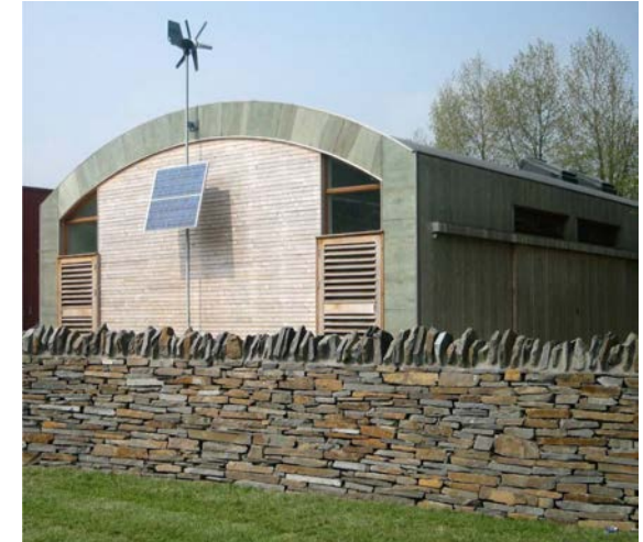
Above: Torfaen Council Eco-Building © White Design
