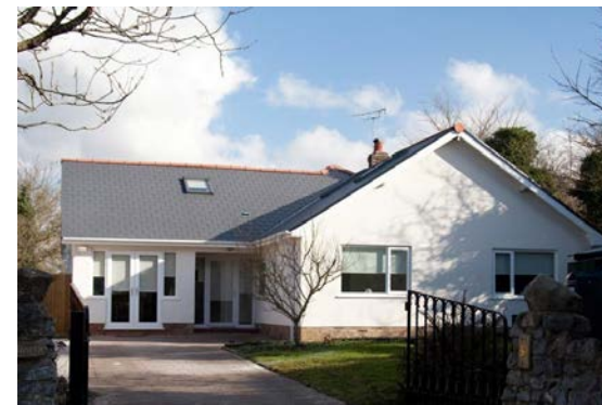
Above: recently renovated adjacent property
