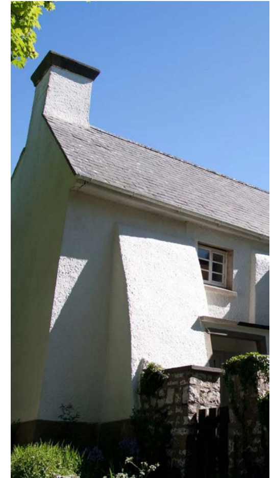
Above: Stone buttress to corner of Great Pitton Farm, Pitton, Rhossili
