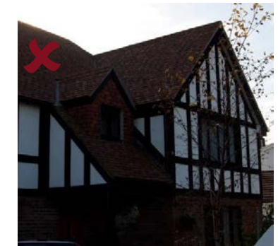
Above: 20th century development with suburban style mock half timbering to upper storey is an inappropriate design response in Gowersually inappropriate
