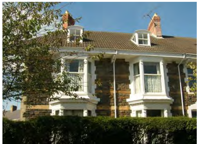
FIGURE 31: These original dormer windows respond to the symmetrical character and pattern of openings without dominating the roof plane
