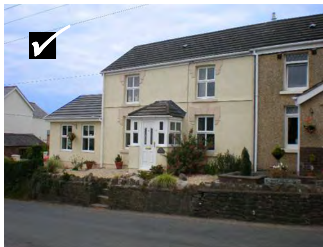
FIGURE 24: This single storey extension successfully incorporates the materials, roof pitch and proportion of windows of the original house
