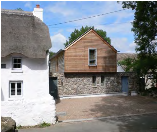
FIGURE 6: Contemporary extension to a thatched cottage, Oxwich (Lord Mayor's Design Awards 2006)
