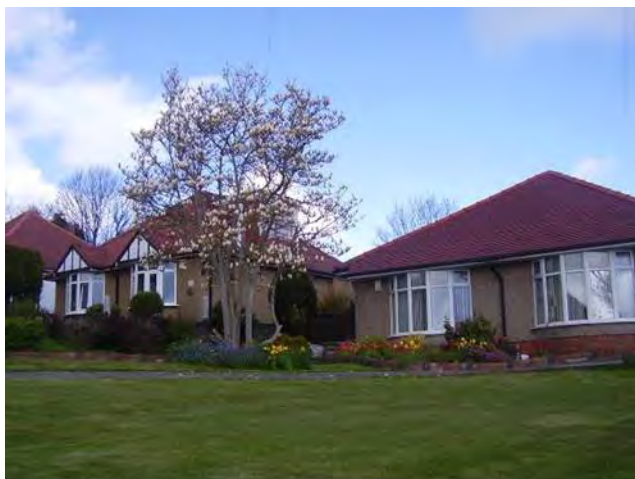
FIGURE 35: Bungalows offer accessible accommodation. Any roof alterations must be carefully considered
