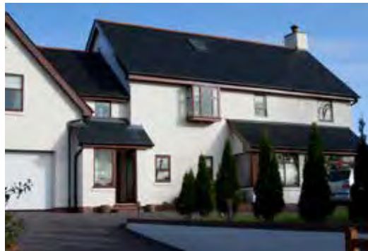
Above: after renovation
