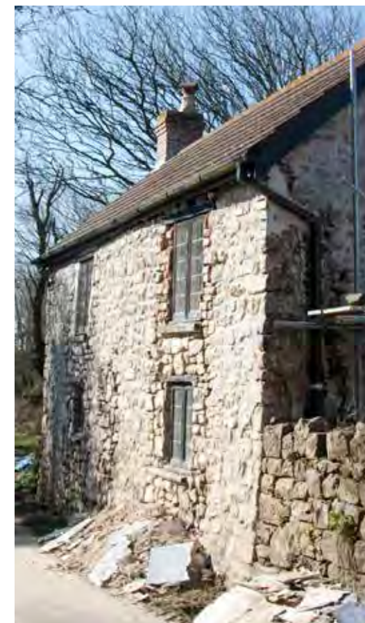
Above: Restoration works in progress, Middleton
