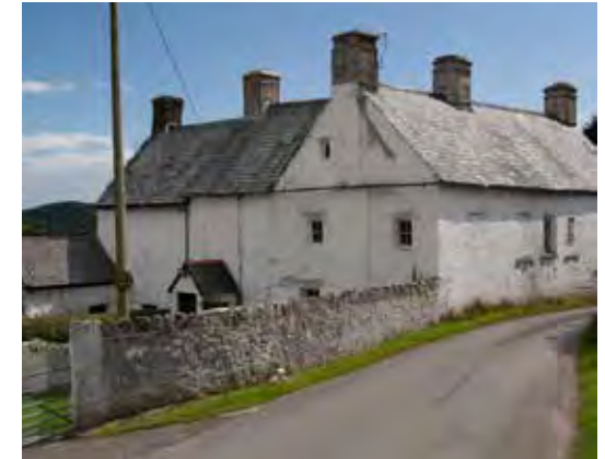
Above: Pitt Farm, above Oxwich is an example of a former small manor house. It does share a number of characteristics of traditional farm houses such as small windows, rendered walls and slated roof
