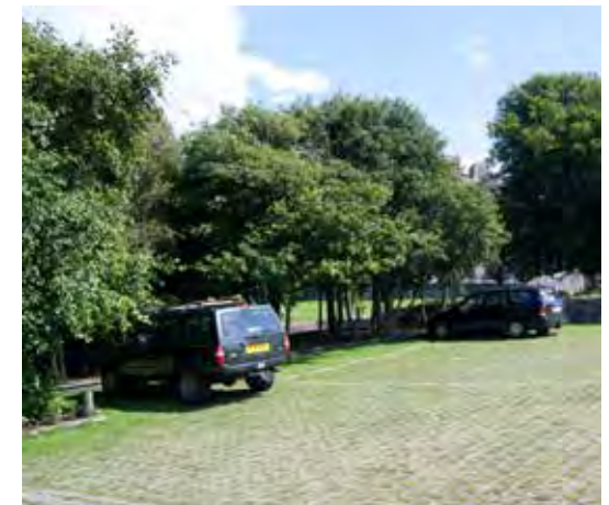
Below: understated reinforced grass provides visually soft parking area at Oxwich Castle
