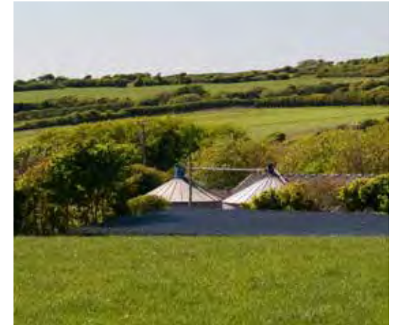
Above: the siting of silo towers within a hollow reduces their visual impact
