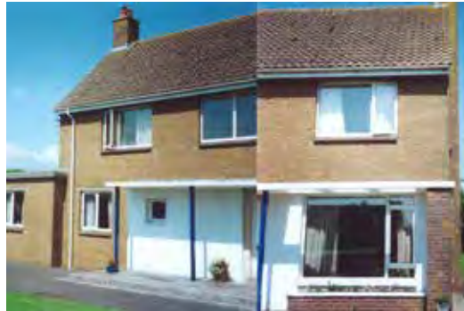
Above: before renovation
