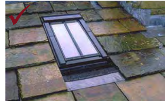
Above: Conservation style rooflight sits flush with roof finish.
