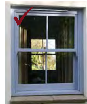
Above: timber sash style painted window
