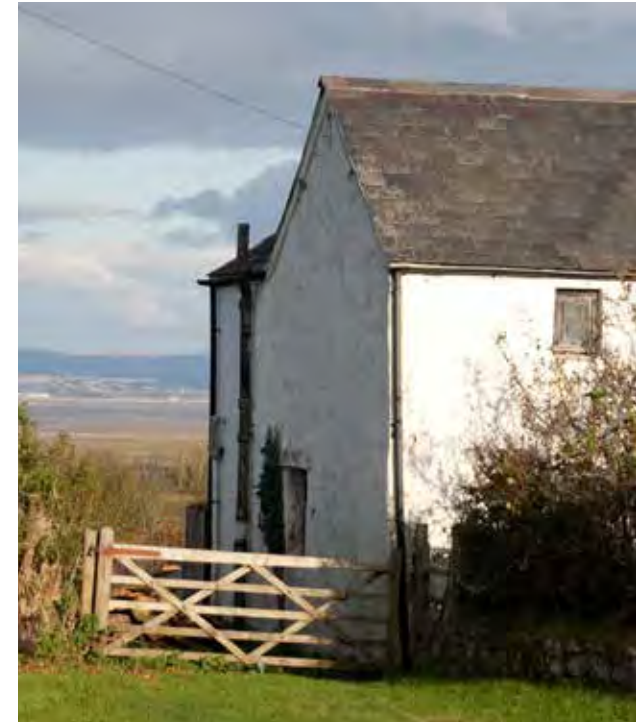
Above and opposite: Properties in Llanmadoc and Oxwich which would benefit from a maintenance regime to retain their character and enhance their surroundings
