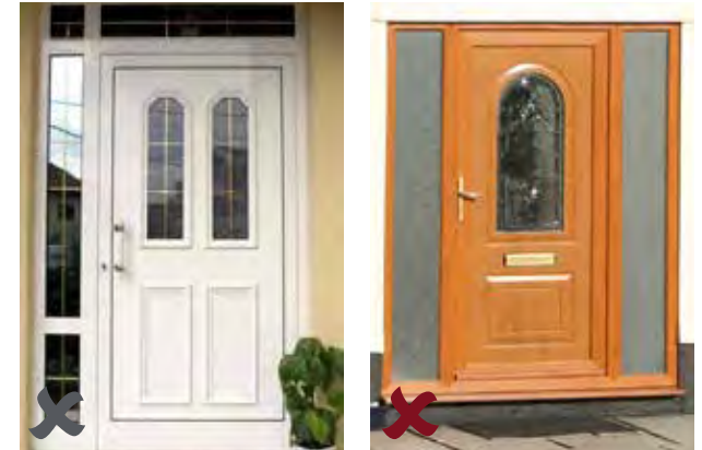
Above: poor examples of doors - use of uPVC and resultant inappropriate style and detail
