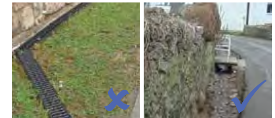
Above: examples of drainage channels and culverts within Gower
