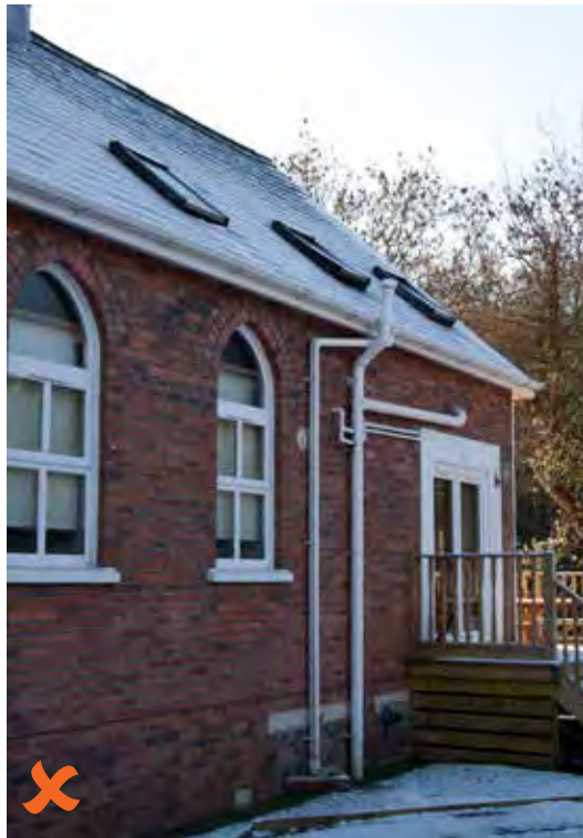
Above: external pipework and timber decking detract from the integrity of this residential chapel conversion
