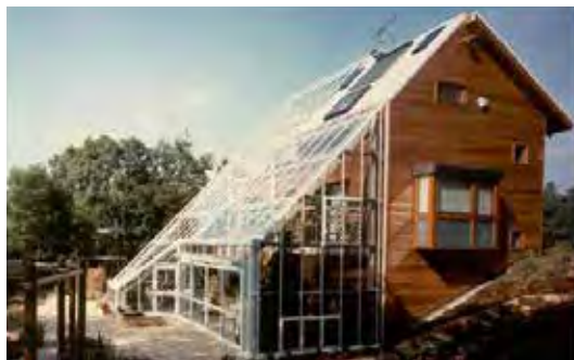
Above: BRE Integer House, Garston Watford
