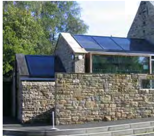
Above: PV installation integral to building design,
