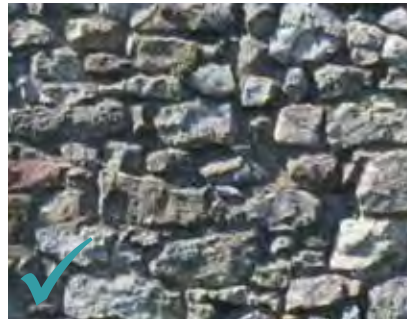
Traditional pointing to stone wall
