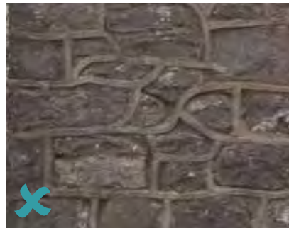
Inappropriate pointing to stone wall
