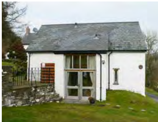
Above: existing openings retained and simply glazed to provide access and daylighting. Brecon Beacons National Park
