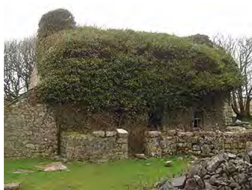
Above: Lack of maintenance can lead to degradation of buildings and landscape
