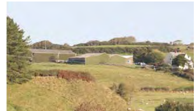
Below: the same buildings treated with a more muted and sympathetic colour are not so prominent in the view
