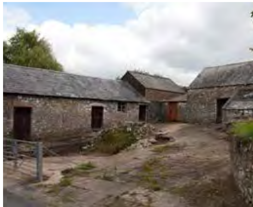
Below: farm buildings used as basis for the preparation of illustrative examples [right]
