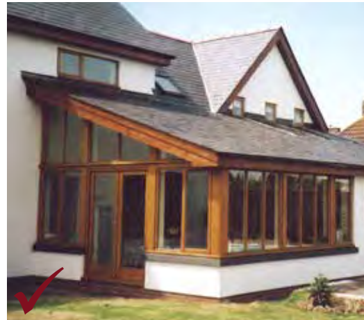
Above: Garden room with timber detailing and slate roof : Southgate
