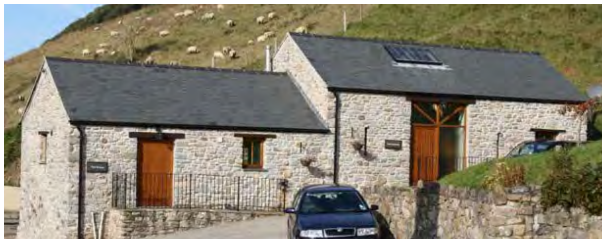
Above: Barn conversion for use as holiday accommodation, Glebe Farm, Cheriton. Utilising existing openings, simple detailing and incorporating level access.
