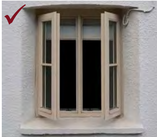
Above: timber opening casement painted window
