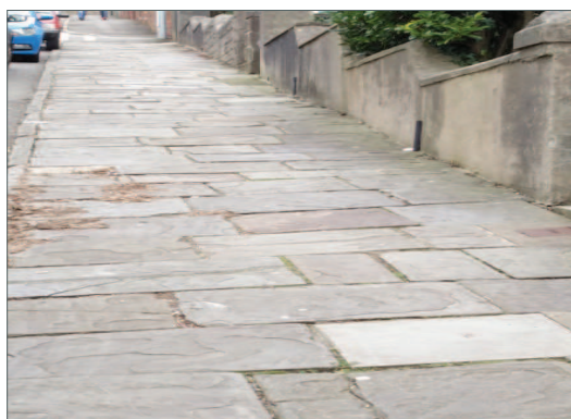
Sandstone Pavement at Cwmdonkin Drive
