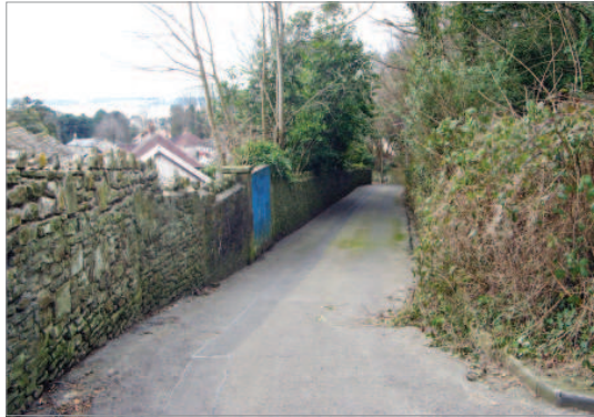
Stone walls in Terrace Road
