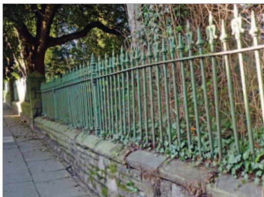
The listed railings around St James's Churchyard
