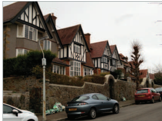
Listed dwellings on north side of Eden Avenue
