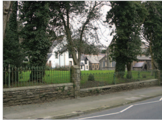
The listed railings around St James's Churchyard
