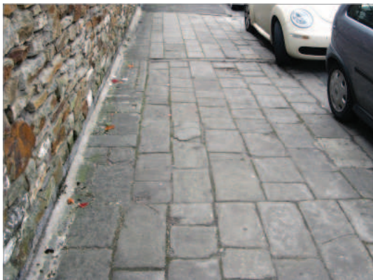
Stone paving in Richmond Road
