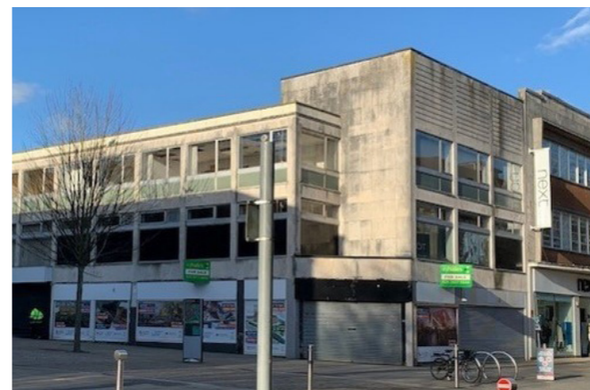
fig 5.37: Portland Road Junction & Next block
