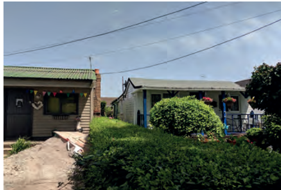
Below: Chalet at Miles Lane
