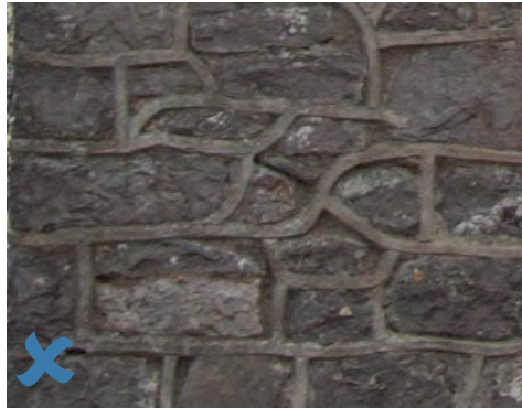
Inappropriate pointing to stone wall
