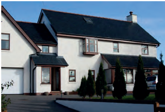
Above: after renovation
