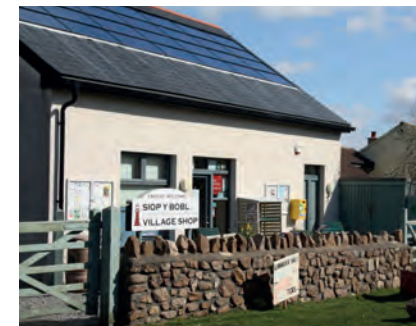
Left: PV installation Llanmadoc
