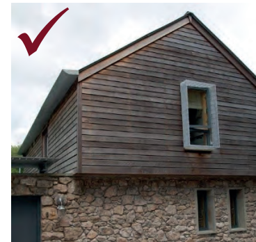
Above: attractive use of timber to upper storey of contemporary extension, with lower storey built in appropriately laid and detailed stonework visually inappropriate
