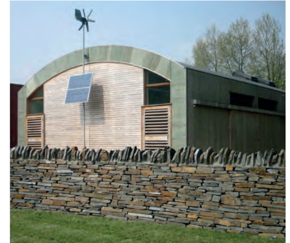
Above: Torfaen Council Eco-Building © White Design
