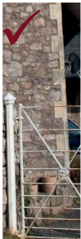
Above: traditional stone quins (left) provide structural support to the corner of the building. This approach has been copied in a more contemporary way using engineering brick (middle) However the use of 'applied' rounded stones (right) is visually inappropriate
