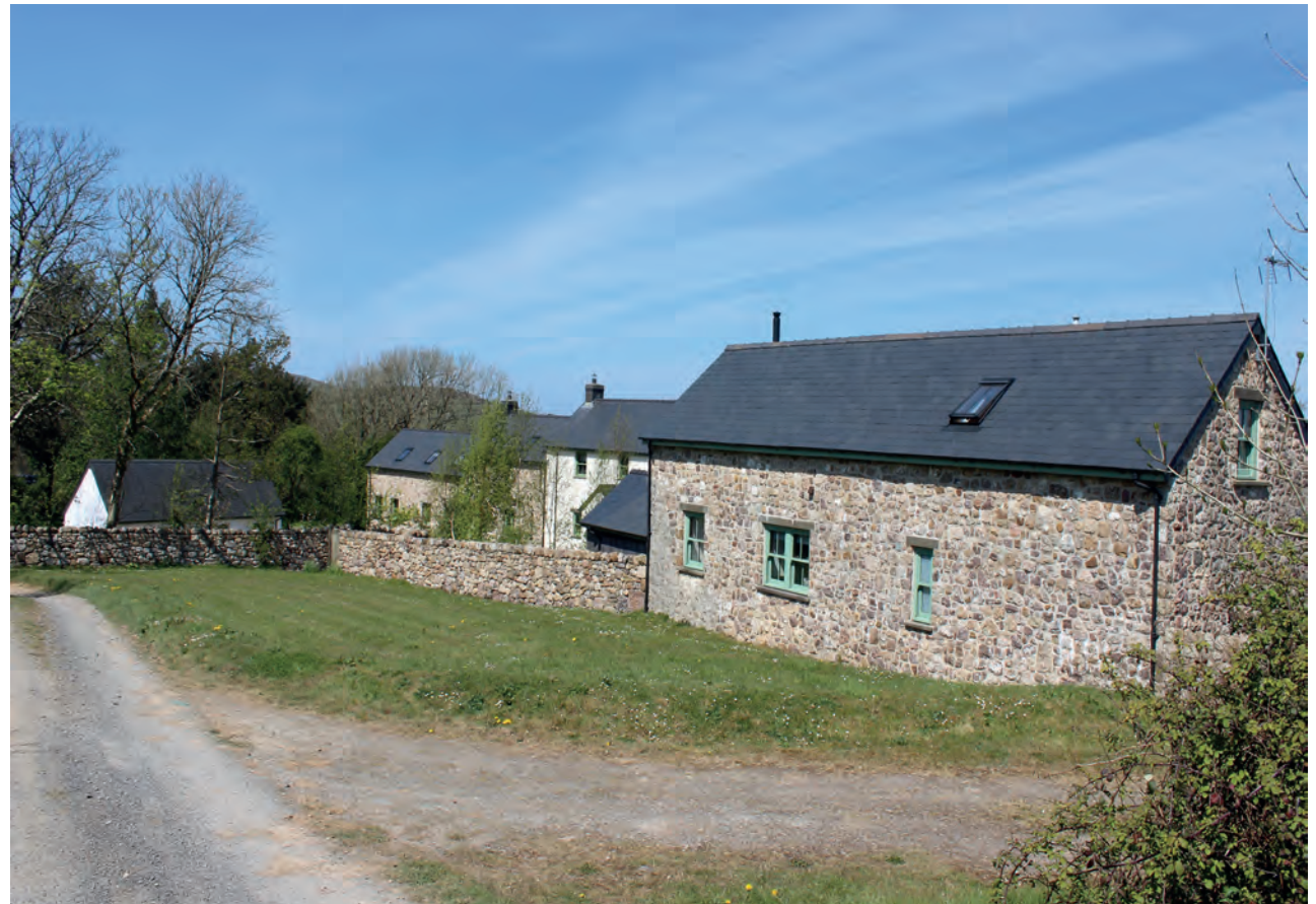
Above: Replacement farmhouse and conversion of outbuildings to provide dwelling house and holiday accommodation, Hill End Farm, Reynoldston. The stone wall, grass verge and planting enhance the development.
