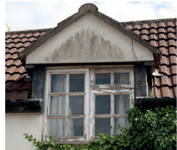
Below: poorly maintained windows can detract from the overall appearance of a building as well as allowing water to penetrate the structure.
