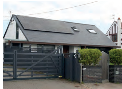
Above: Photovoltaics to roof, Southgate
