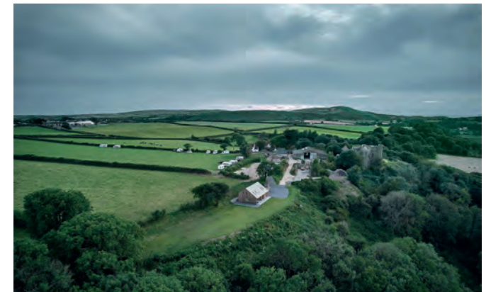
Above: New rural enterprise dwelling at Weobley Castle Farm, Gower, lying adjacent to the working farm. The house is modest in scale and footprint, with a simple pitched roof design, timber clad walls and roof clad in sheeting. The design draws on the rural agricultural vernacular and conforms with the 'contemporary vernacular' approach set out in this Placemaking Guidance document. As a result the proposed new house is subservient in the countryside and viewed as part of the existing established farm complex. Images @ Raum Architects
