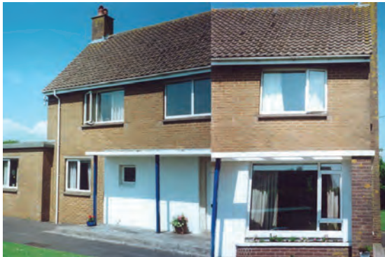
Above: before renovation
