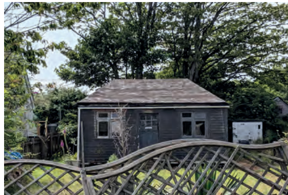
Below: Chalet at Sandy Lane
