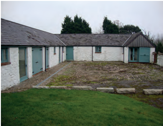
Above: Existing openings retained and simply glazed to provide access and daylighting. Home Farm, Penrice.
