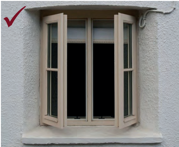
Above: timber opening casement painted window
