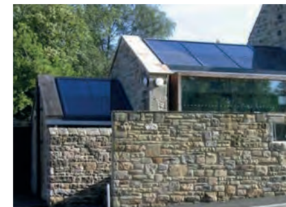
Left: PV installation integral to building design
