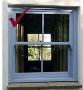
Left: timber sash style painted window
