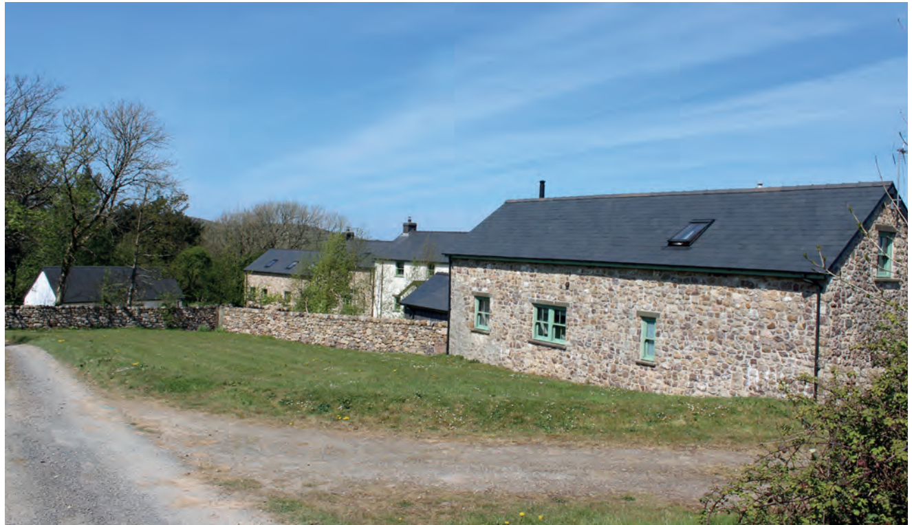
Above: Replacement farmhouse and renovated outbuildings, Hillend Farm, Gower
