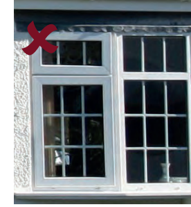
Left: uPVC opening and fixed casement window with overly wide frames
