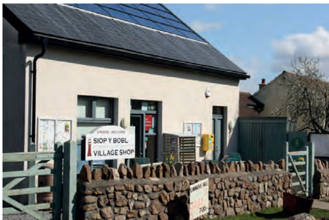
Above: Llanmadoc Village Shop
