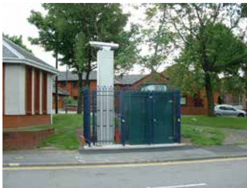
Photo 2 - St Thomas DOAS Receiver Station
