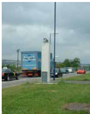
Photo 1 - St Thomas DOAS Transmitter
