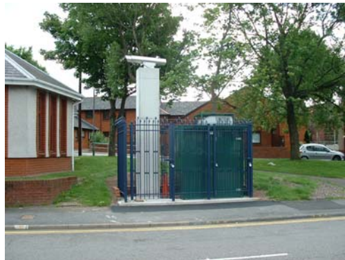
Photo 2 - St Thomas DOAS Receiver Station
